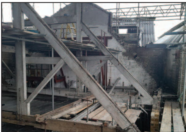
Roof of Frogmore Mill
